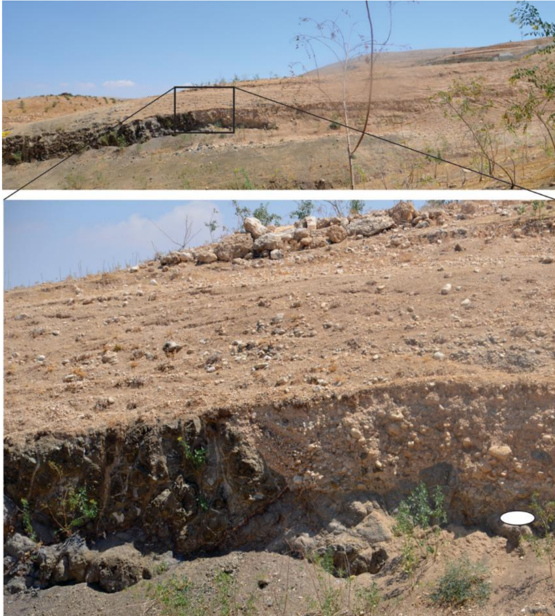
Fig. 12: Site 457, looking East, Dawqara Fm?. Note the erosion of the basalt layer. The white ellipse points to the giant core recovered in situ .
